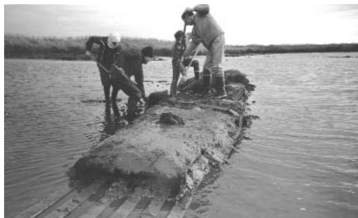
Building floating islets for ducks and terns. (Guérande salinas, 1986)
