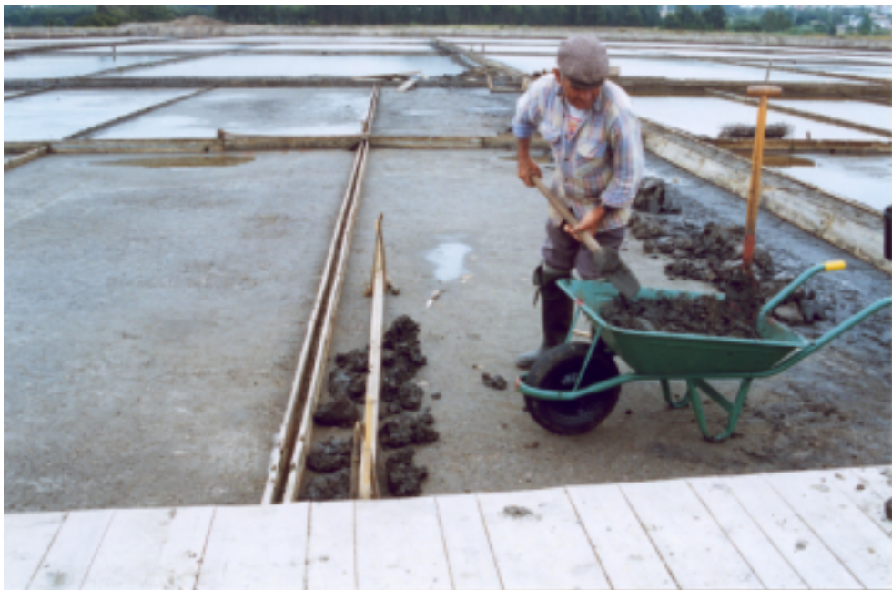
Figure 24 - Replacing a caneiro
