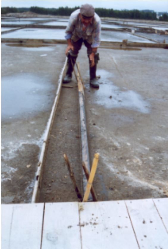
Figure 21 - a) Placing the guide to build up the maracha and b) filling in
