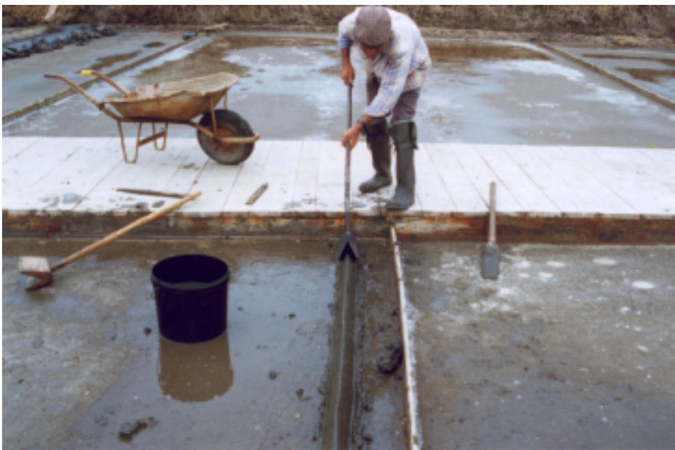
Figure 22 - Shaping with the mould
