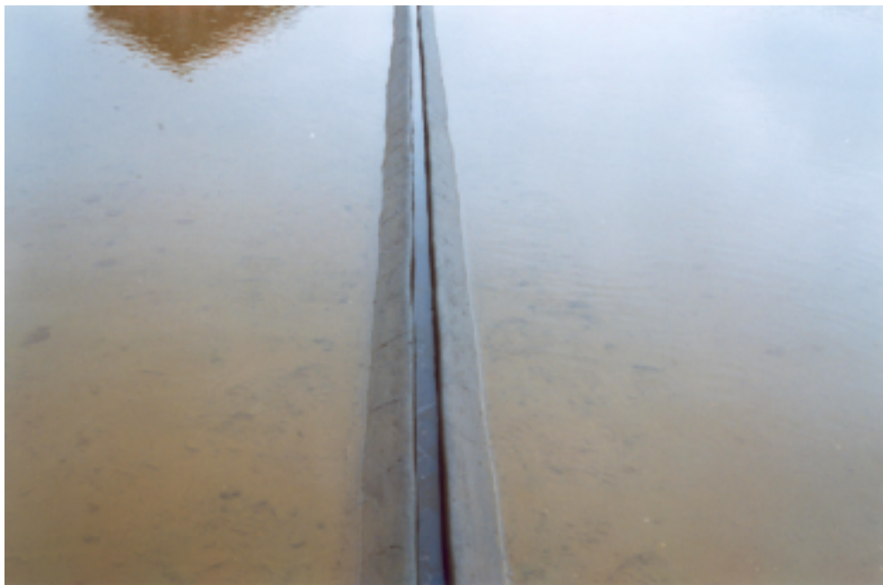
Figure 26 - A completed caneiro
