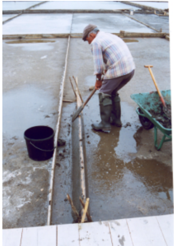
Figure 21 - a) Placing the guide to build up the maracha and b) filling in
