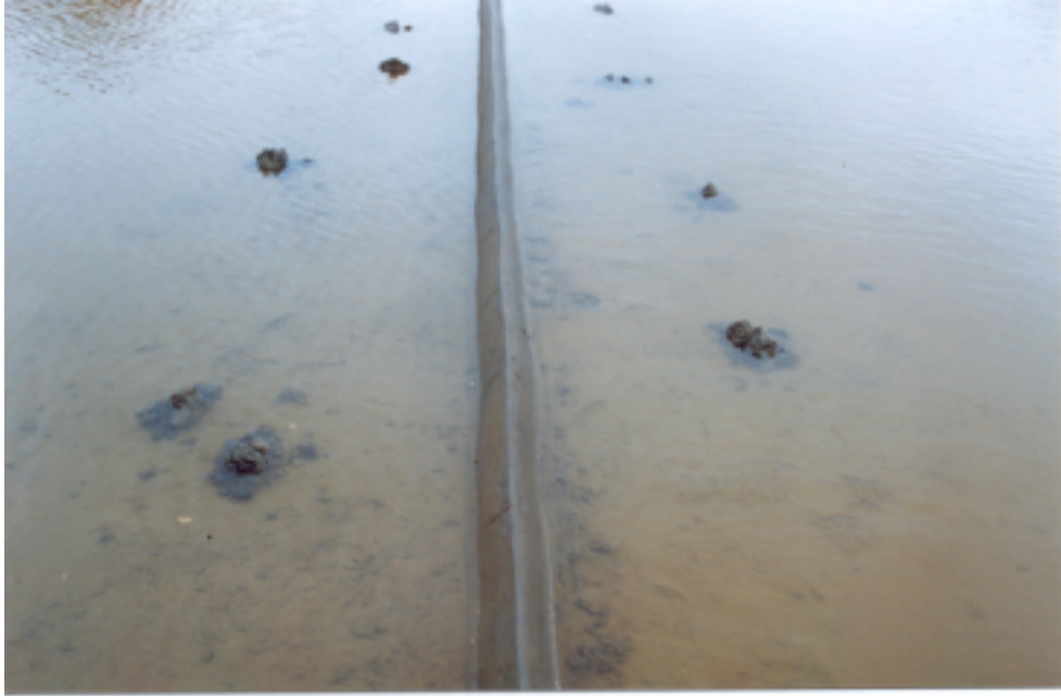
Figure 23 - A completed maracha , replacing a wooden one
