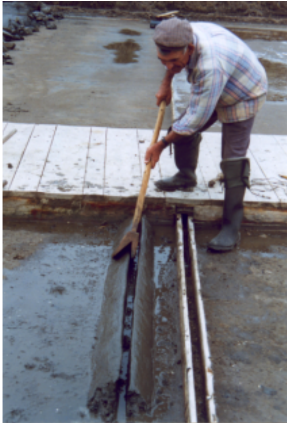
Figure 25 - Shaping with the mould
