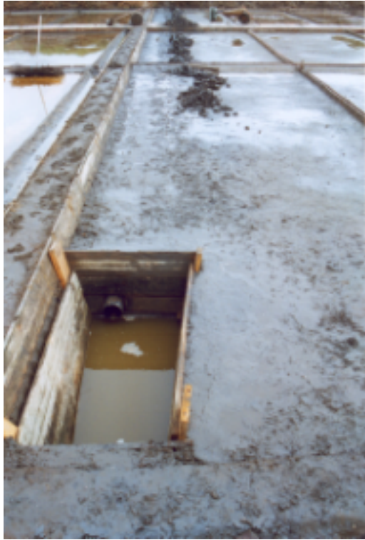
Figure 30 - Rebuilding the poço for a pump
