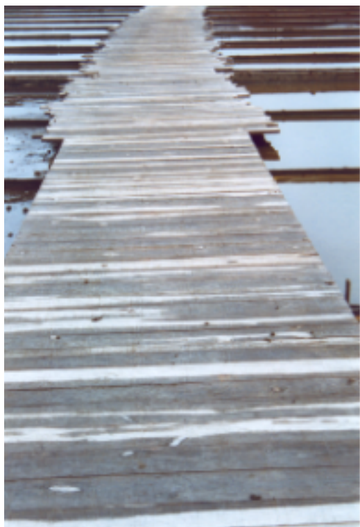
Figura 27 - Replacement of boards on the silha
