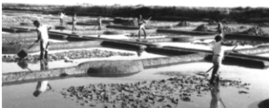
Figure 3 - Restoration work at La Grande Ségestine saltworks
