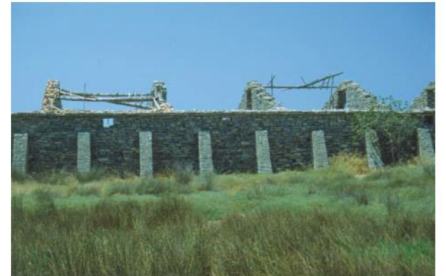
Warehouse for storing salt in Samos, Greece
